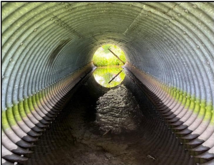
Looking south through barrel
