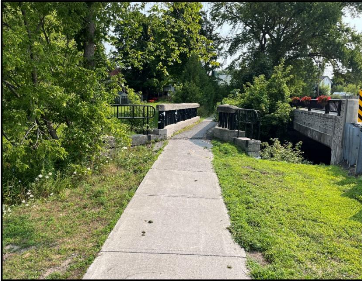
Walkway looking east
