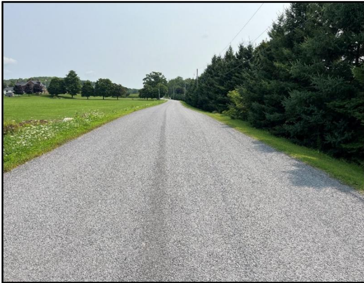
Roadway looking east
