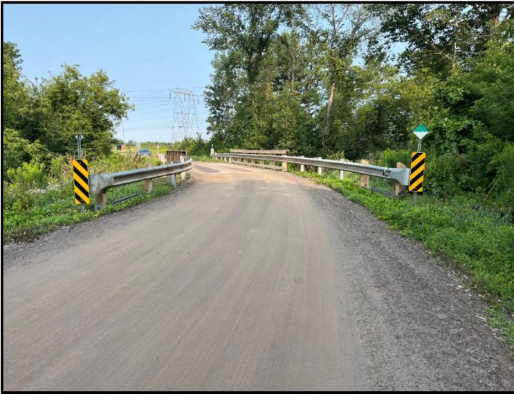
Roadway looking west
